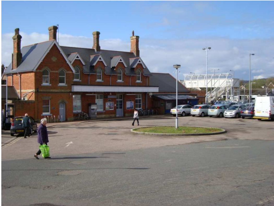
Borough Green Station
